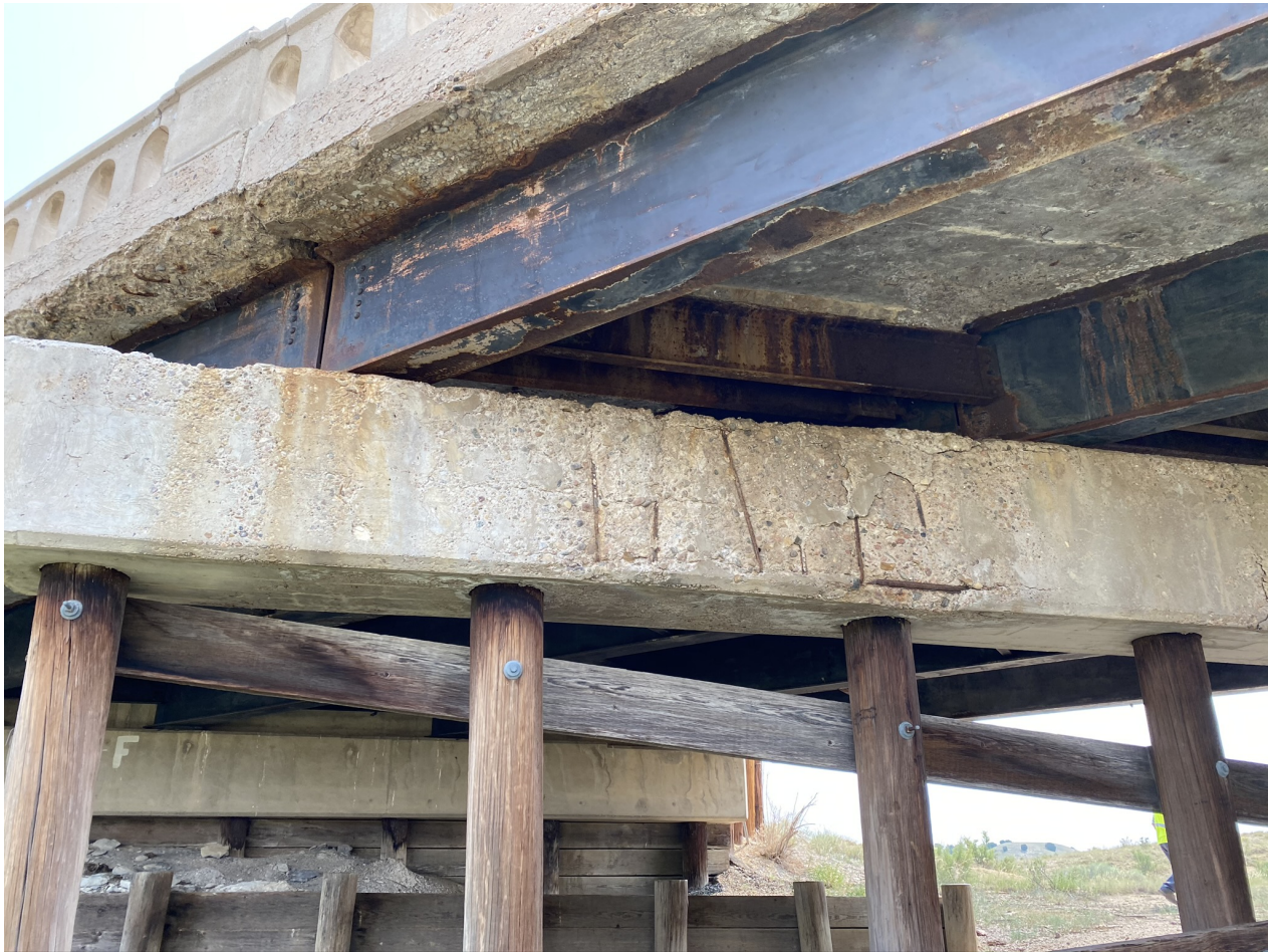
Picture 2 - Pier, Overhang, Deck, Girders
